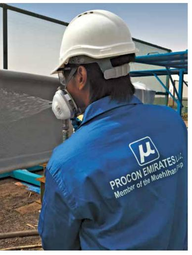
Application of fire protection on steel construction
